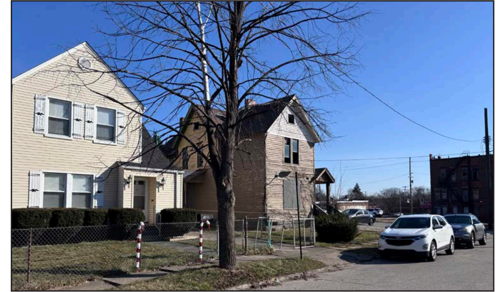
VIEW FROM GARDEN AVE LOOKING EAST
